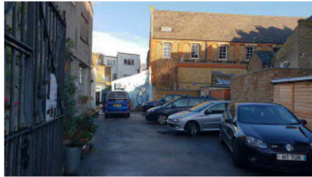
View from Blackwater Court towards the Unit 8
